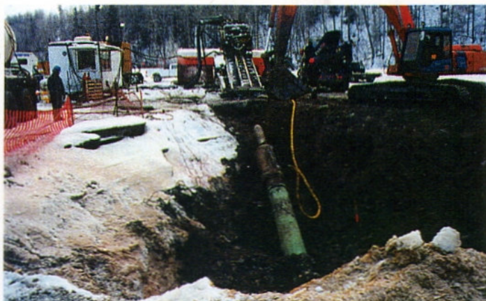
A 180-ft (55-m) surface casing is extracted on the entry side.
